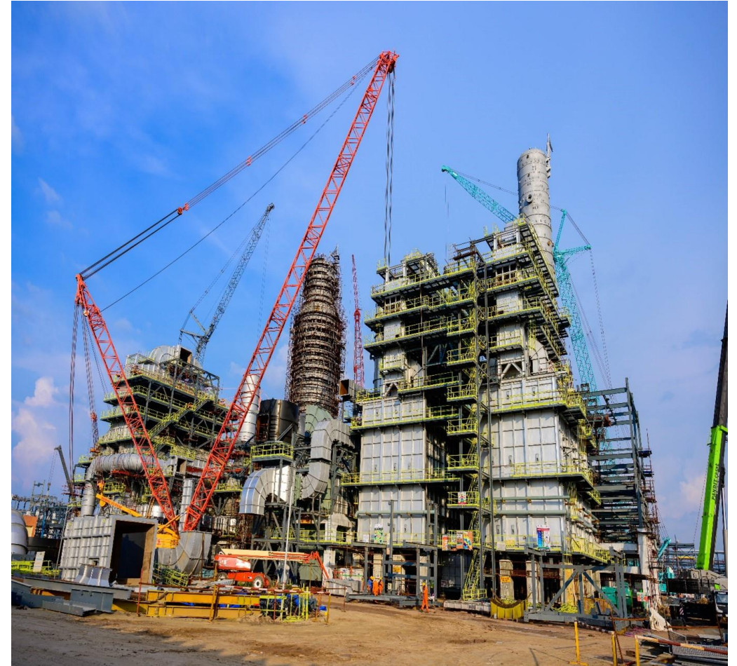
HRRL Project, Rajasthan
