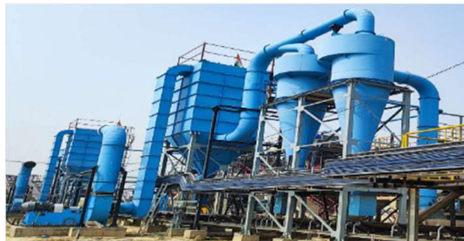
CBG Plant at Budaun- Milling Section
